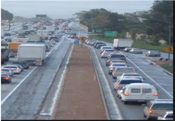
1.a Merging of two entry Ramps on A highway
