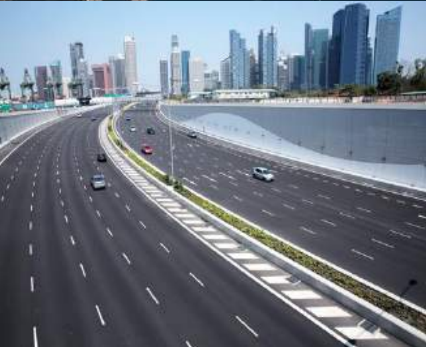
Marina Coastal Expressway (2016) 12 lanes of capacity regulated by ERP and static ITS systems with peak period congestion and fall in level of service
