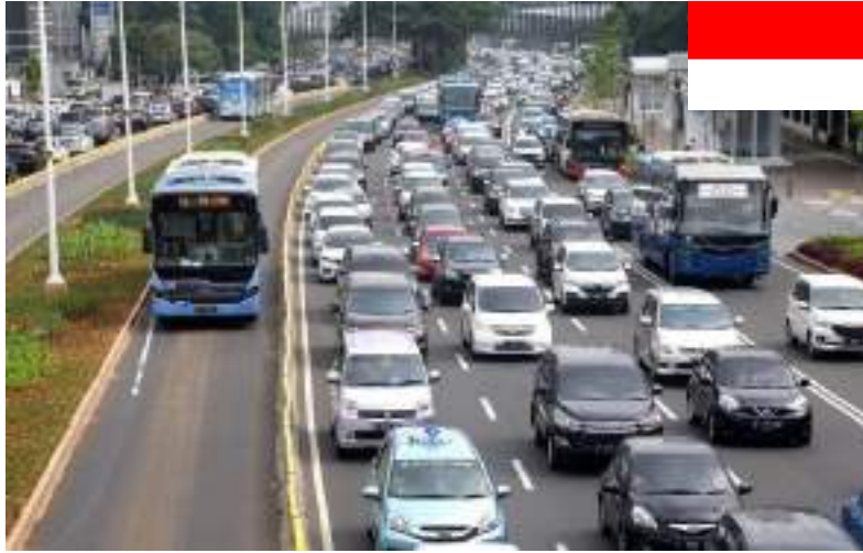
Highway in parallel with an exclusive ROW lane on Jl. Sudirman, South Jakarta
