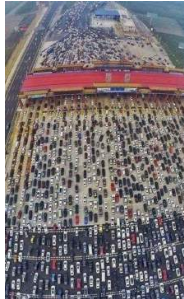
Toll plaza merged from 25 lanes to 4 lanes in Beijing - Hebei section
